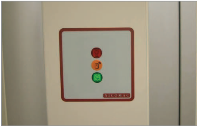
Flush interface with HPL and interlock indicator light.
